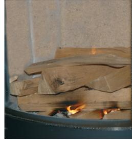
2. Fully open the "side" air control. Light the firelighters and leave the door slightly ajar to allow air to enter and the fire to establish.
